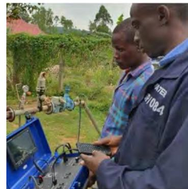
*Inspection and regeneration of boreholes by the static plant team*
